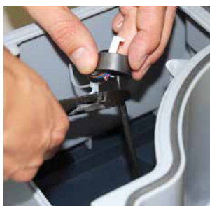
17. Cut the electric wire.
