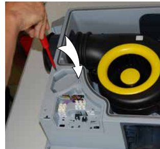
28. Fix the electrical case on the fan case (4 screws).
