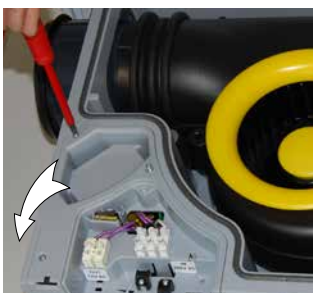
4. Unscrew (4 screws) the electrical case.
