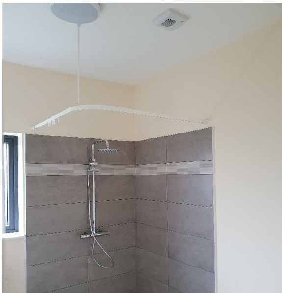
Demand controlled exhaust units were used in the bathrooms and Kitchen. They provide the right amount of exhaust ventilation and are connected to the V4A fan
